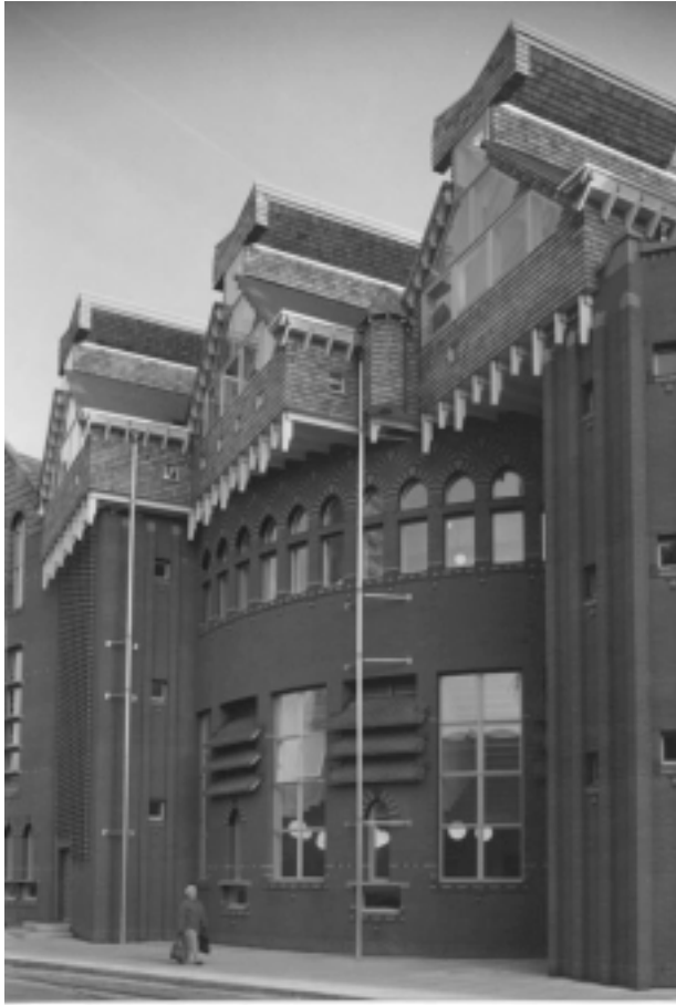
The Queens Building on the DeMontfort University campus makes optimal use of natural daylight and natural ventilation to reduce energy requirements
